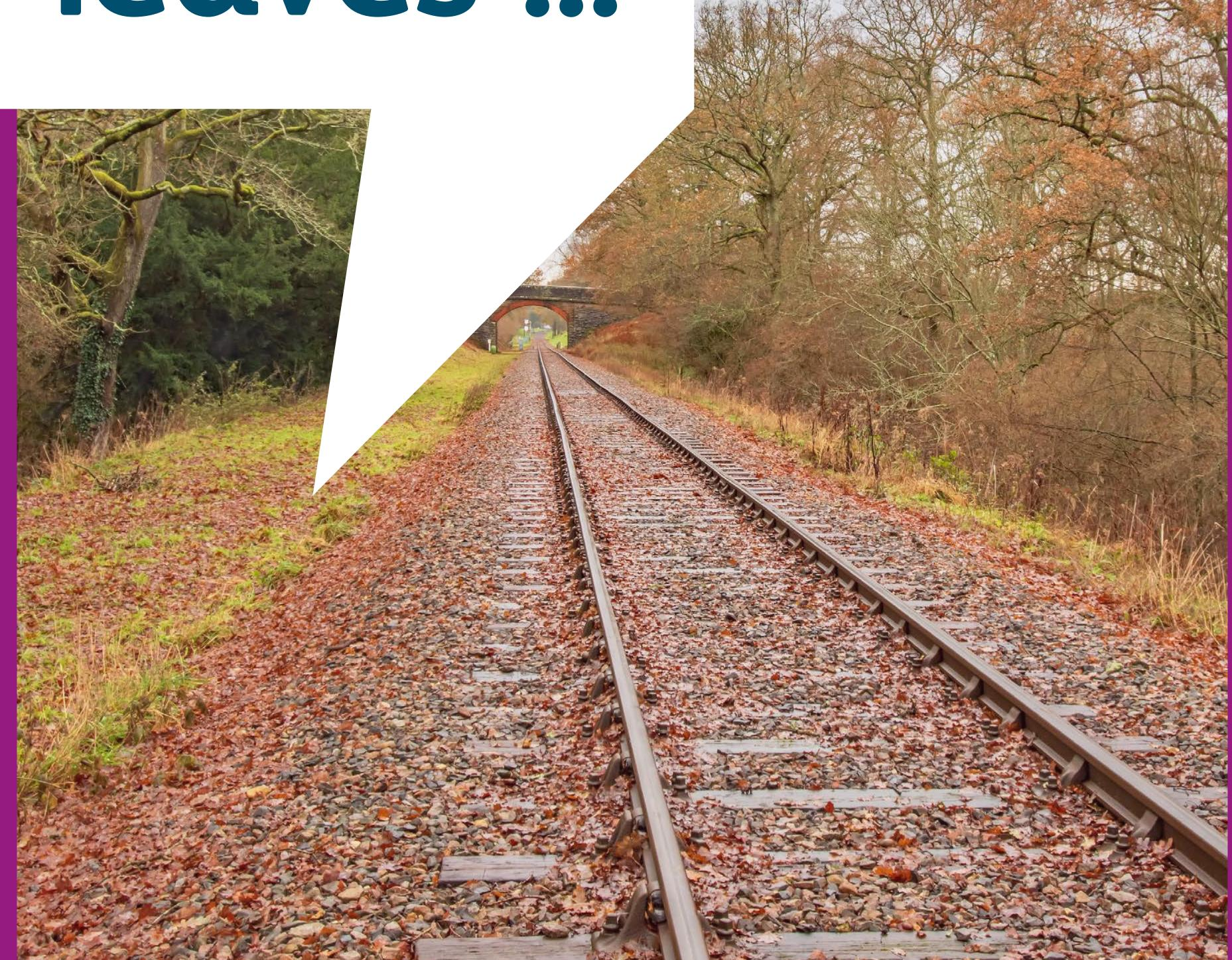
In fact, a build-up of leaves is more likely to stick to the rails. The heat and weight of trains passing over the leaves bakes them into a slippery layer.
