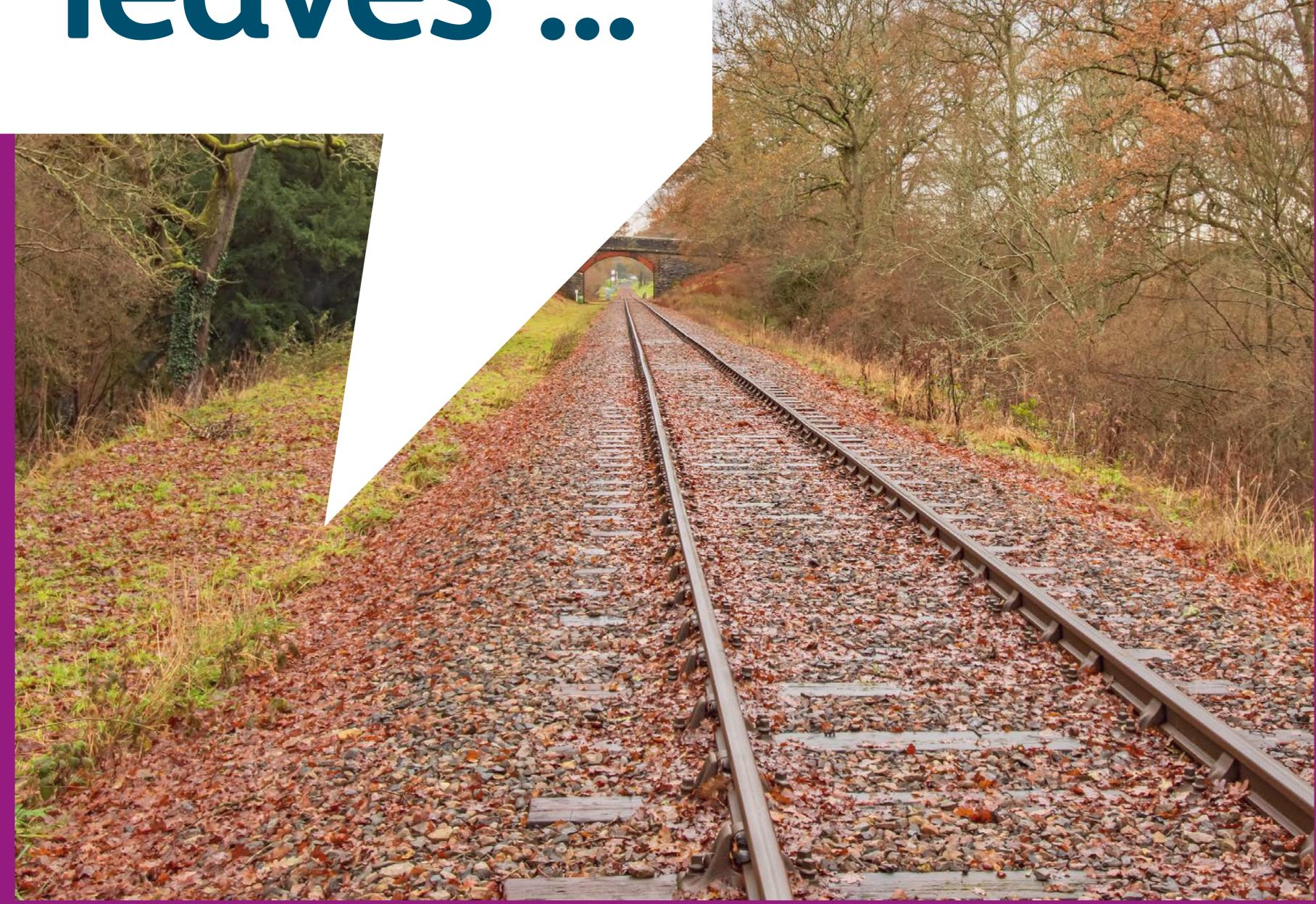
In fact, a build-up of leaves is more likely to stick to the rails. The heat and weight of trains passing over the leaves bakes them into a slippery layer.
