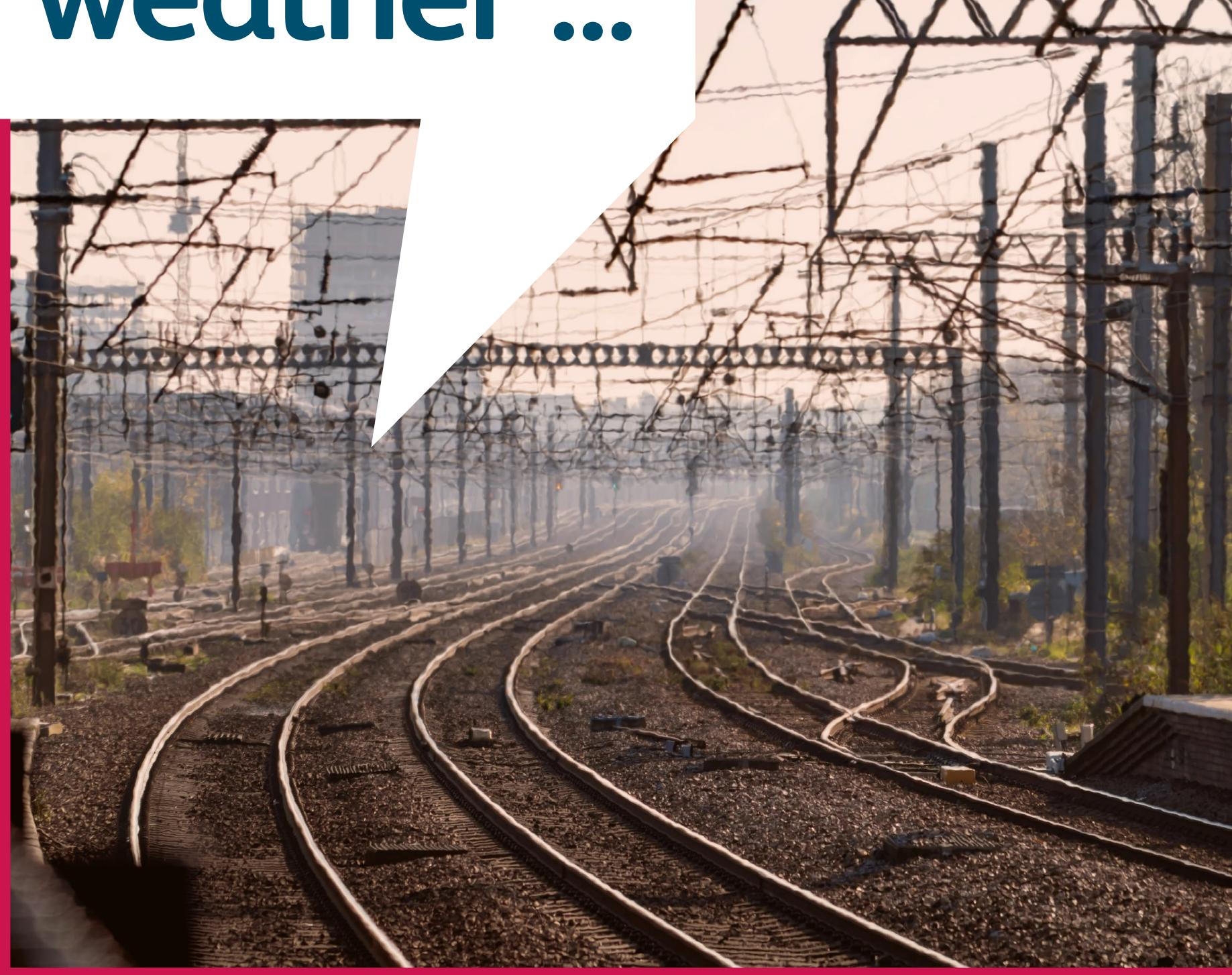
In fact, hot weather can cause the overhead lines to expand and sag. To avoid damaging the lines, trains must travel more slowly than normal.
